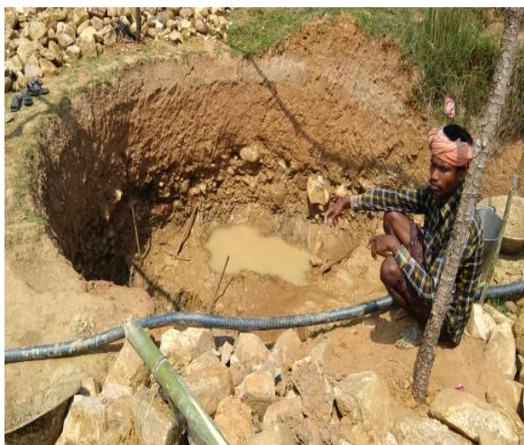
Figure 7.2: Creating Dug Well on Individual Land at Hinjilicut Block in Ganjam
